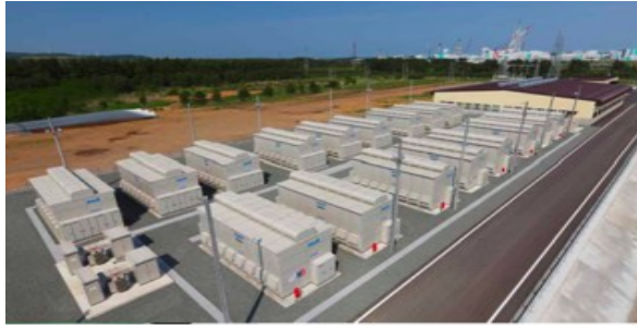
Figure 6. Storage technologies can increase utilization of intermittent resources like wind energy. These sodium sulfide batteries have been integrated into a wind farm in northern Japan.
